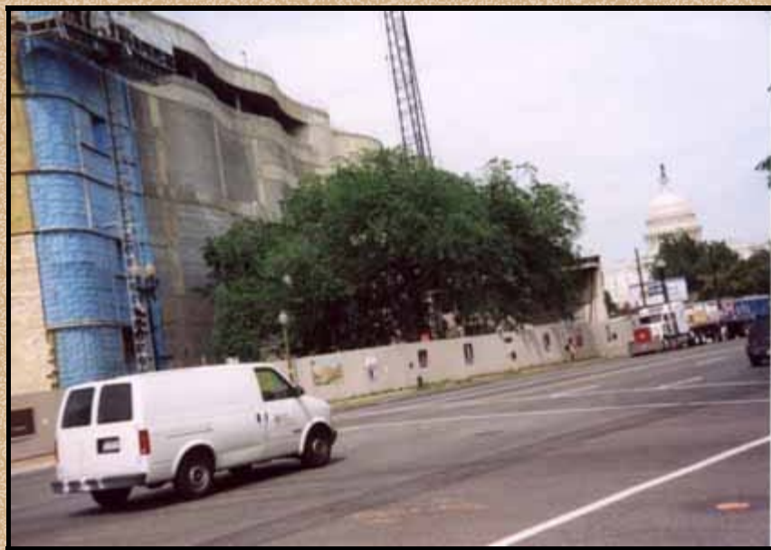
LAB FILM S104:531 South Wall at Independence Avenue
